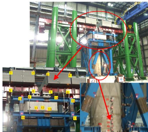
Fig. 2. Photograph of the real size bridge model on the shaking table. The diameter of the bridge pier was 1800mm, and weight of the specimen was 1500tons.
